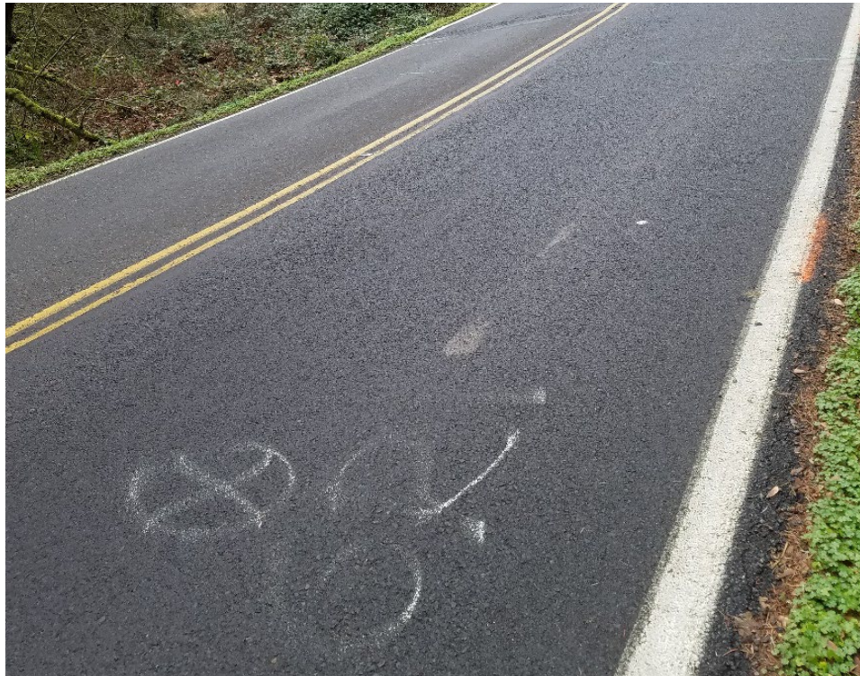
Core B-5 (SW 105 th Ave., STA 23+86, FWD #29 NB)
