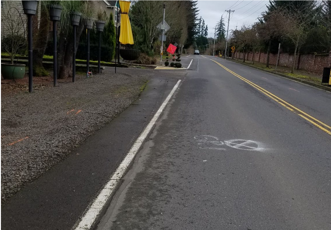
Core B-4 (SW 108 th Ave., STA 12+89, FWD #5 NB)
