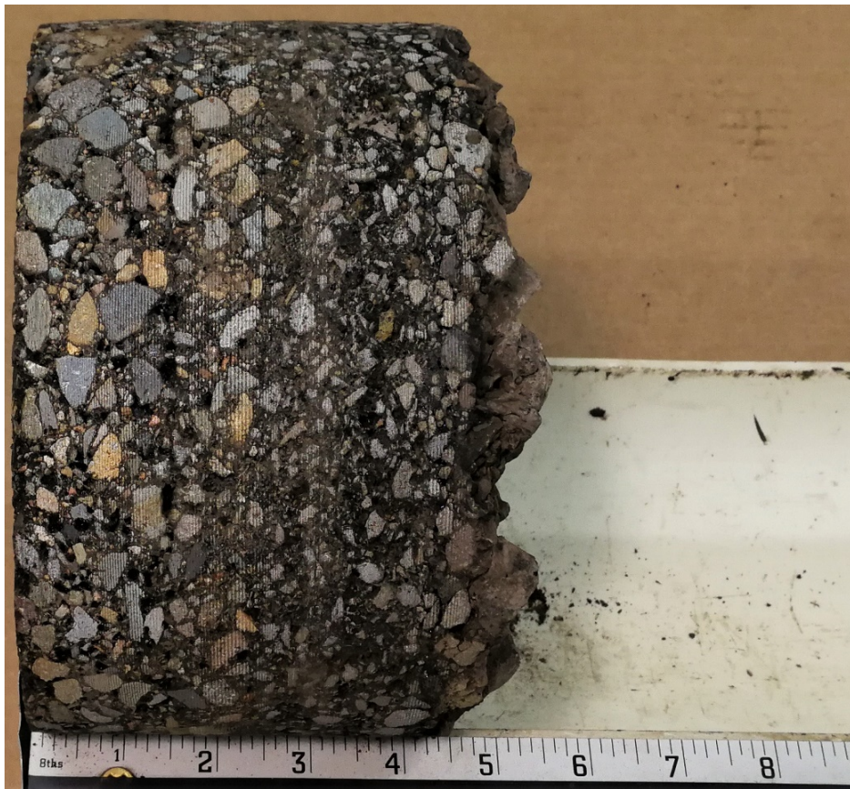
B-2 (Pavement Core Sample, 4.75 in.)
