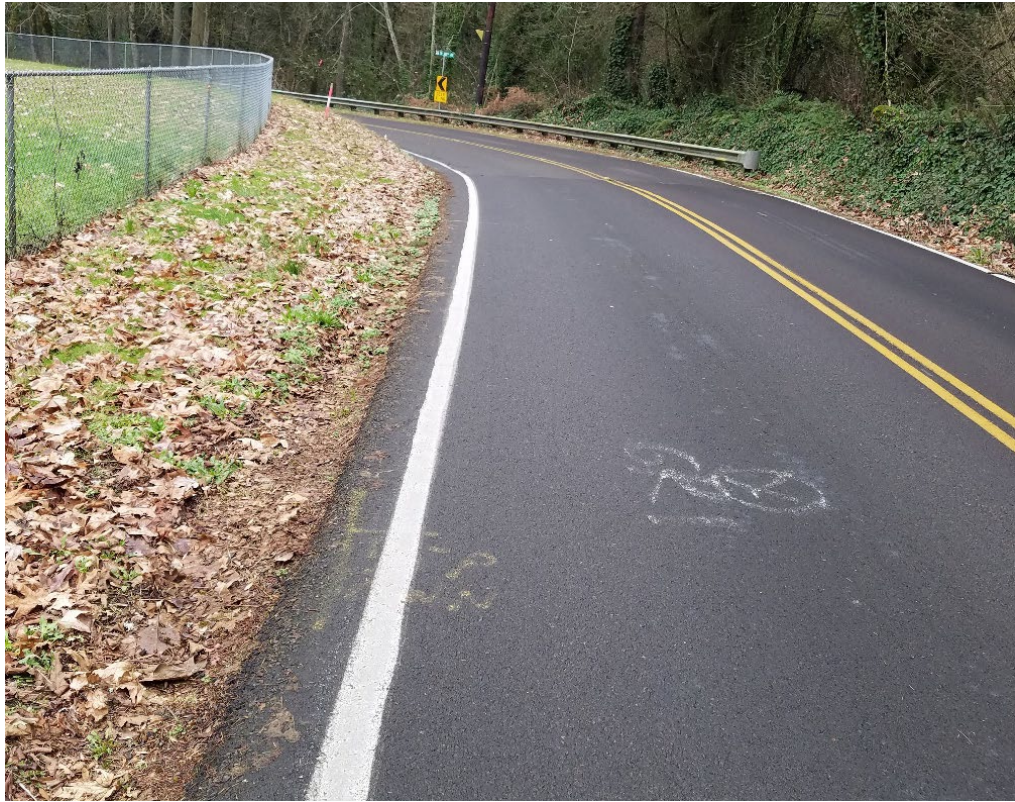
Core B-3 (SW Blake St., STA 19+78, FWD #20 NB)
